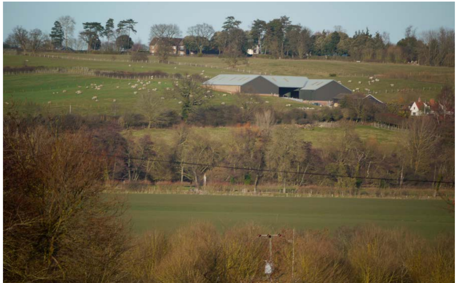
Highly reflective roofing material
